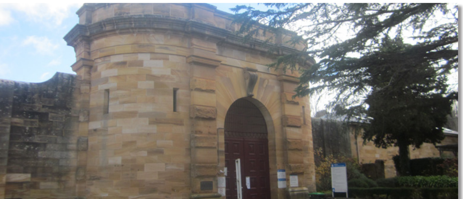
Works at Berrima Gaol were the refurbishment of the facility to become operational after being closed for a number of years. Works at the gaol included hydraulic services, electrical services, painting throughout and an upgrade of the facility security system.
